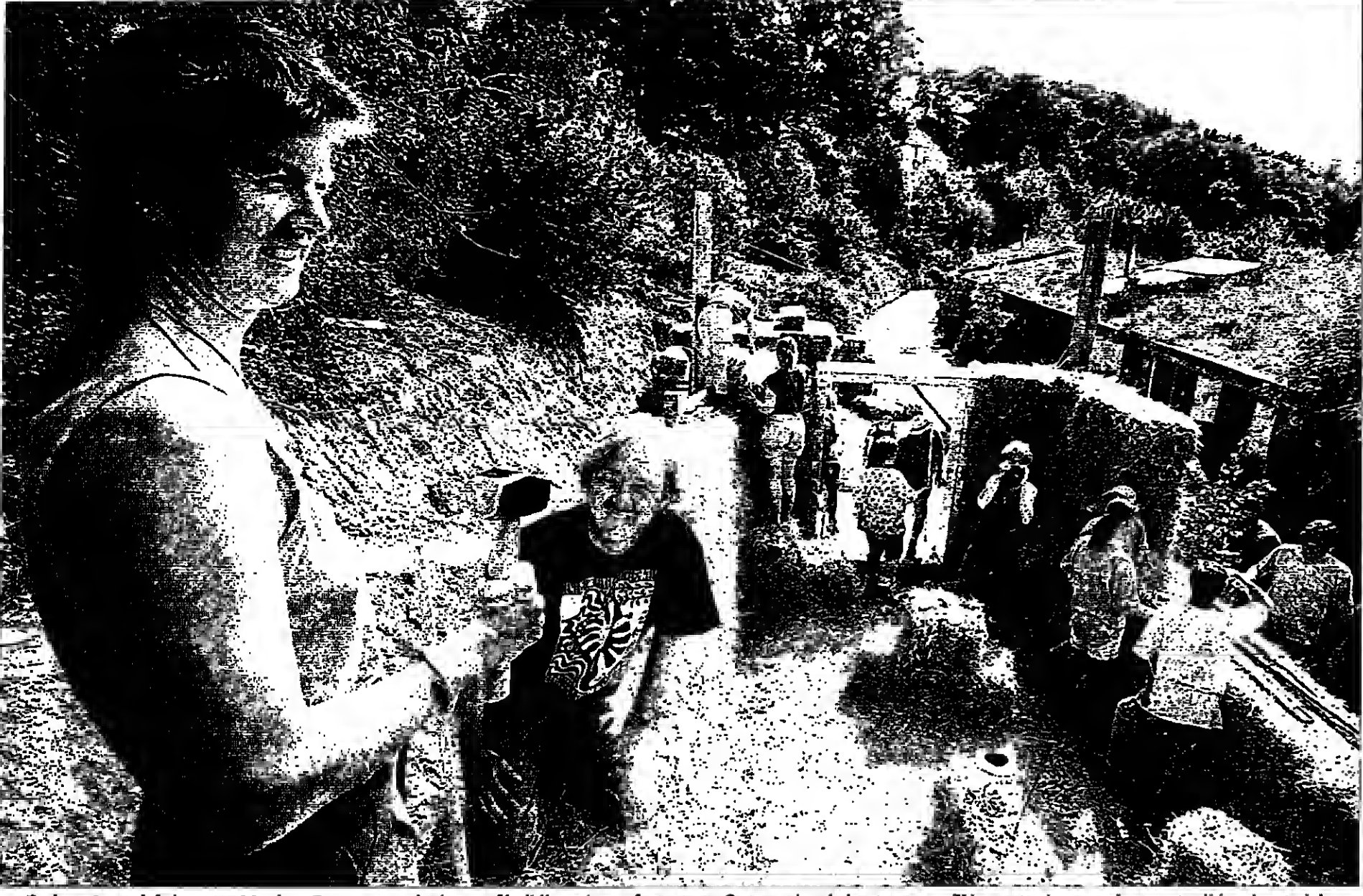
Barbara Jones, left, instructs Matthew Brace, centre, in the art of building a house from straw. Once rendered, the structure will be as sturdy as any in more traditional materials
